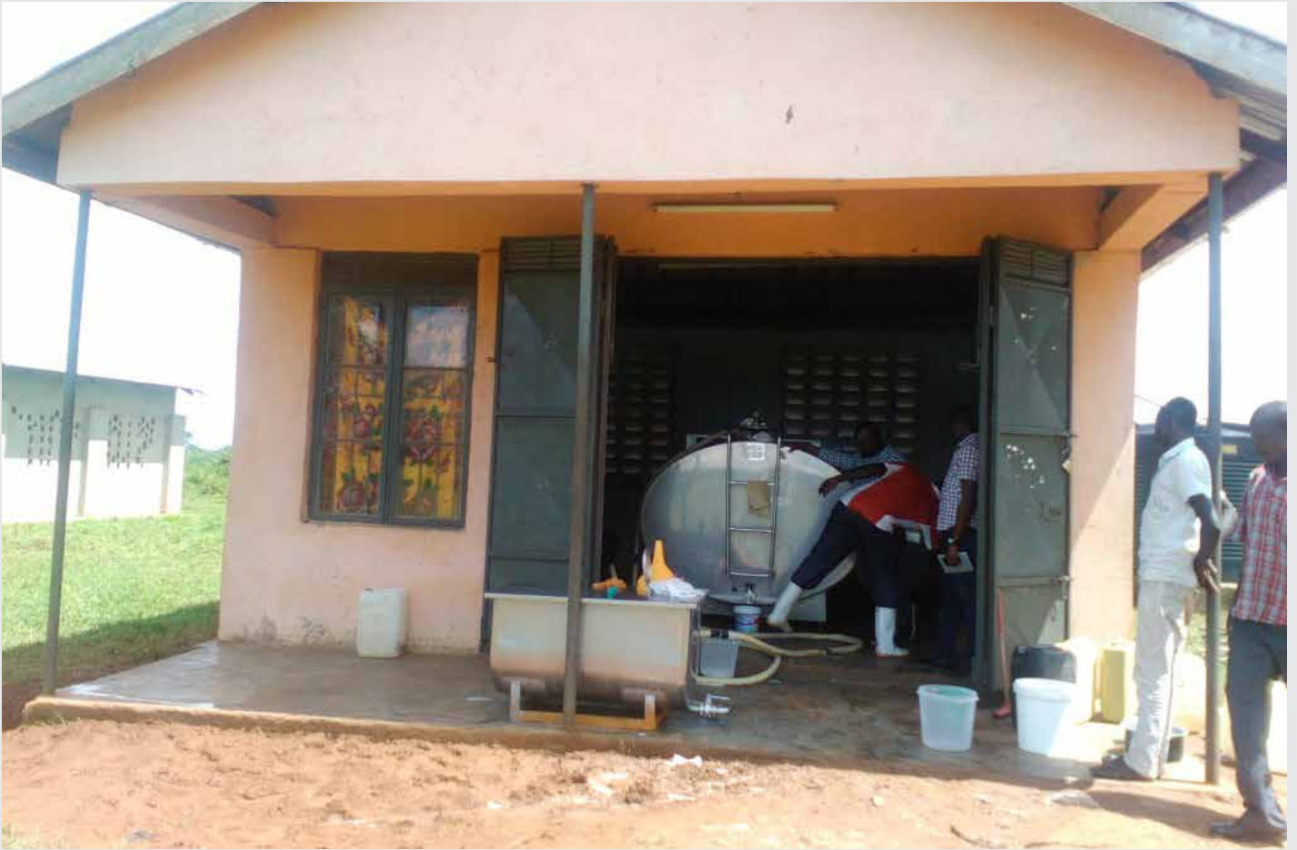
Buyende dairy cooperative chilling plant
